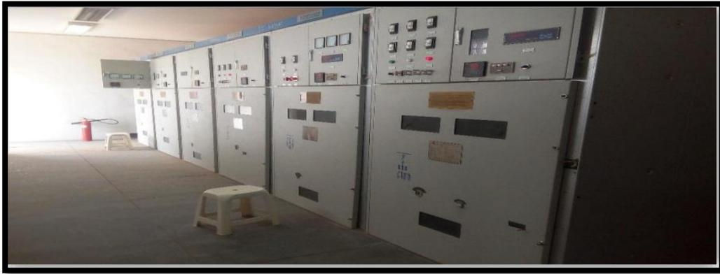
**Figure I.12 : Arrive sonal gaz 16MVA.**
