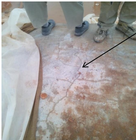
Photo 2.57. Fissures apparentes.
