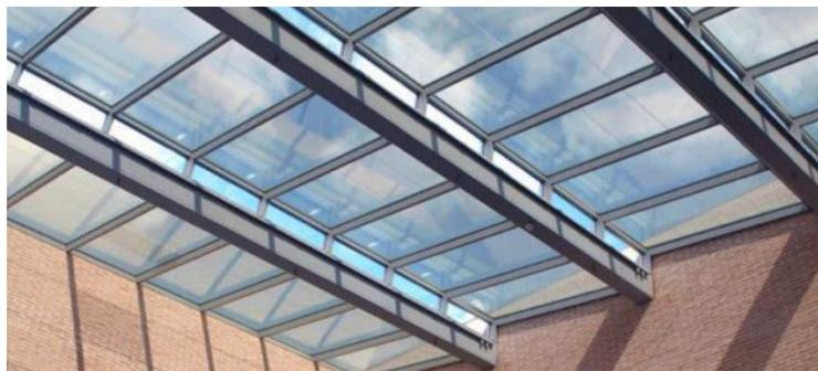
***Figure.35*** Vitrage photovoltaïque transparente [32].
