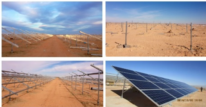
FIGURE 3.4 – Montage des supports
