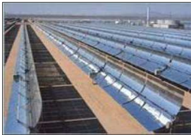
Figure I.1: centrale solaires thermique [7]
