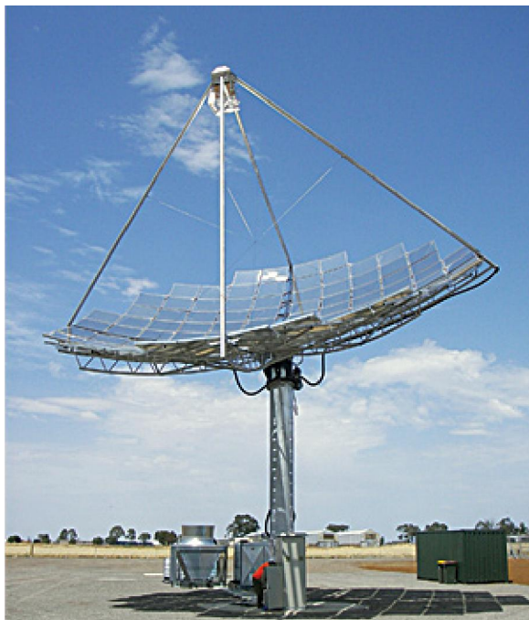
Fig. 2.48 - Système HCPV Solar Systems. 40 kWc DC (STC). Photo [102].
