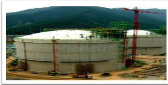
**Figure I.18.**reservoir a double integrité
