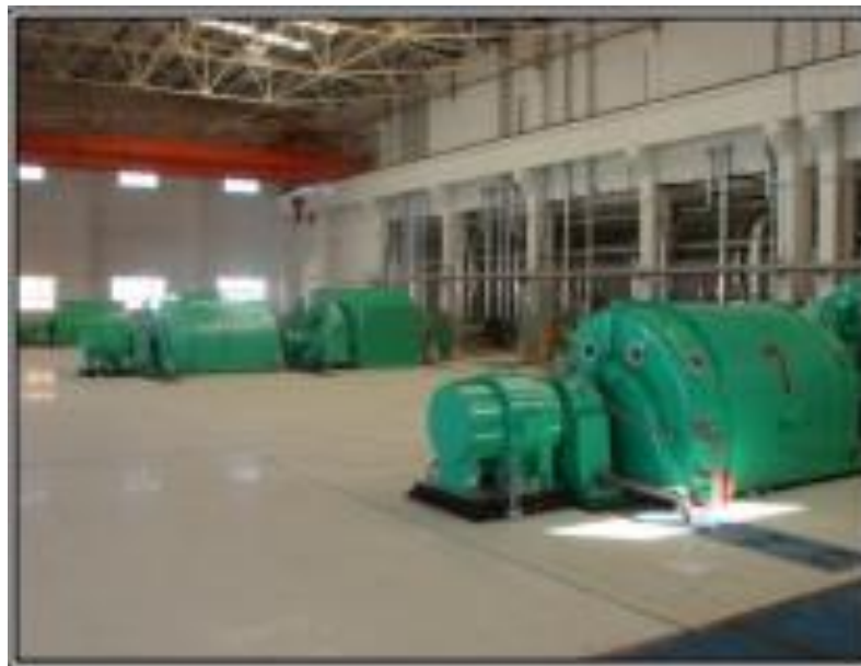
Figure I.61 Turbo generator
