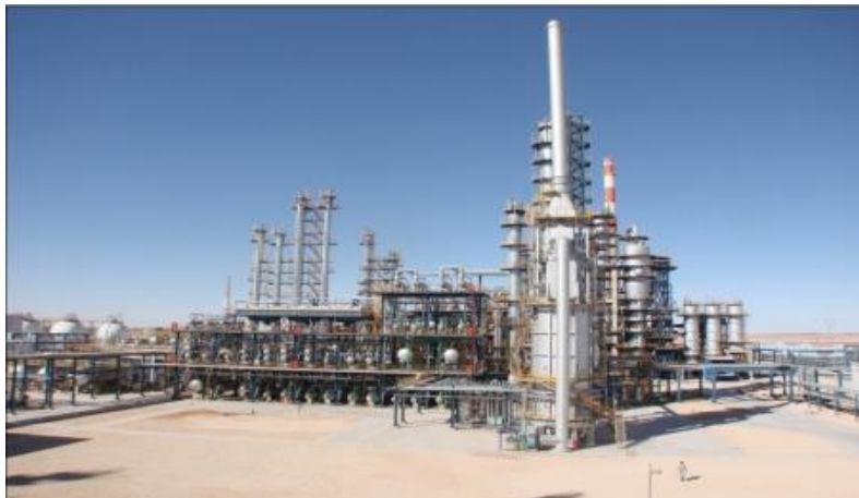
Figure I.21 View of the atmospheric distillation unit
