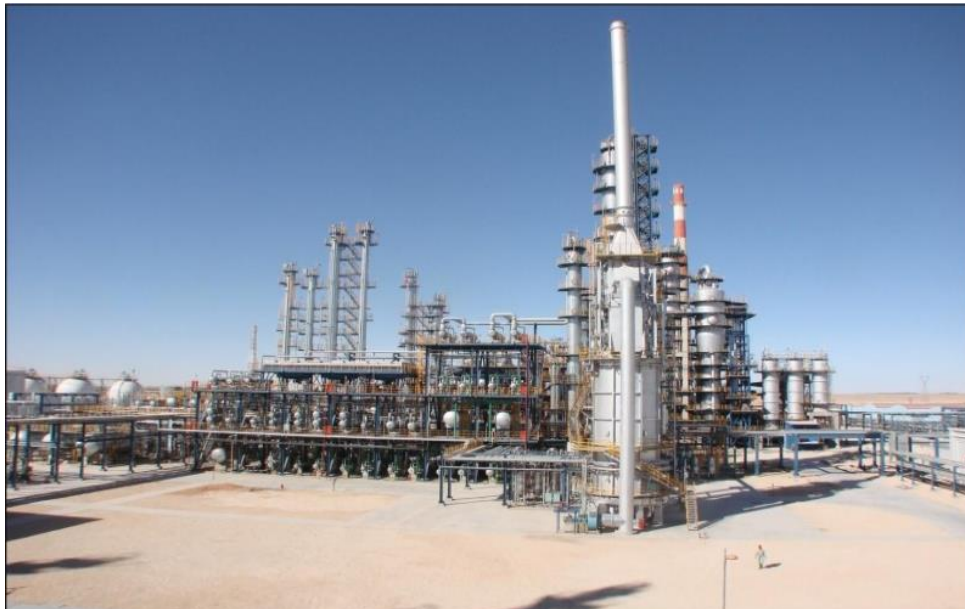
Figure I.66 View of the atmospheric distillation unit
