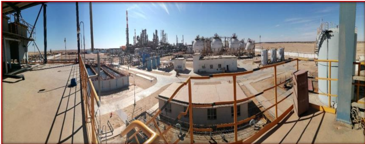
Figure I.1 THE ADRAR REFINERY
