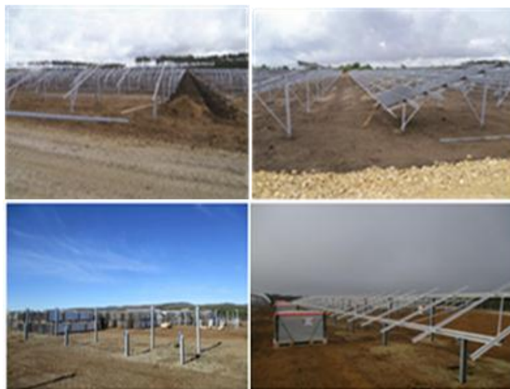
Figure.II.4 : Montage des supports.
