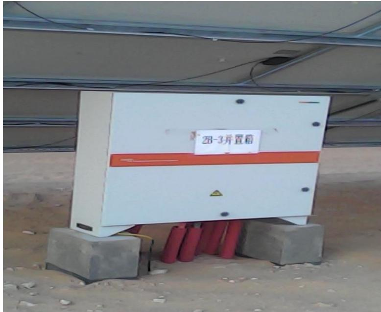
**Figure III-13:** Boite de raccordement
