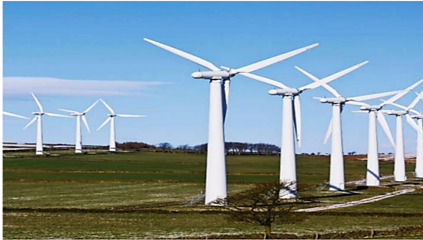
Figure I.3: Wind Turbines [GSH 17].
