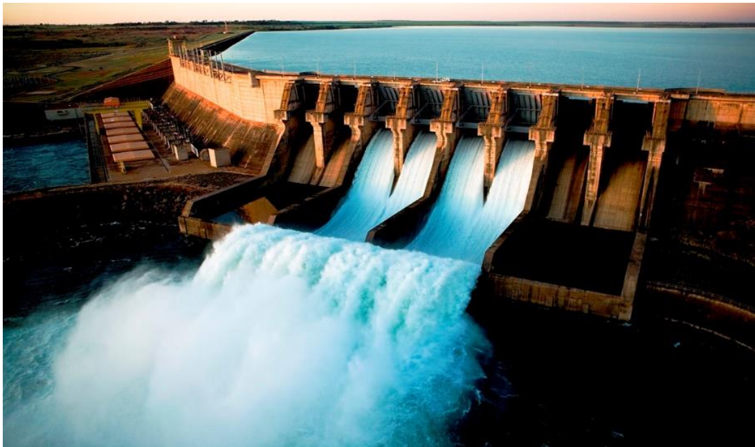
Figure 1.1: Construction of Hydropower Project
