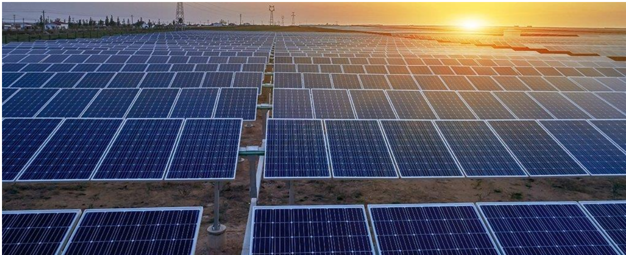
Figure 1.4 Photovoltaic Solar energy panels.
