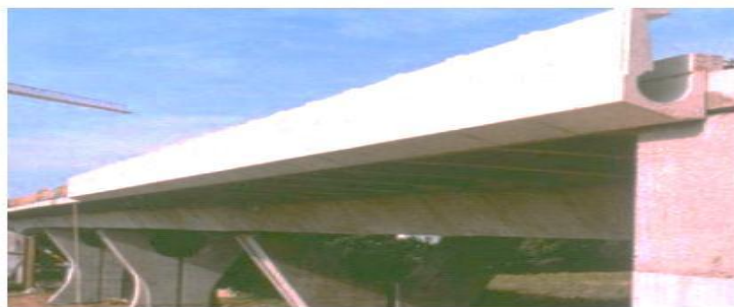
Figure II.15 : Exemple de corniche-canneveau [16]
