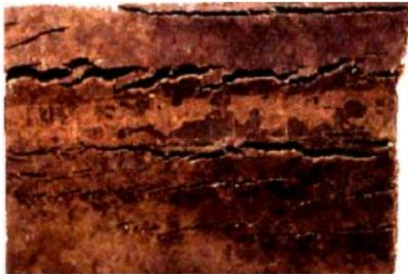
Figure 10:Fissures de CSC [2]
