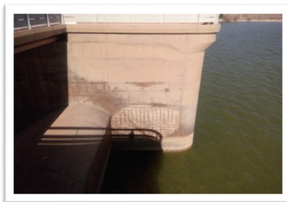
photo II. 2: Barrage Djorf Torba (partie Amont) [18]
