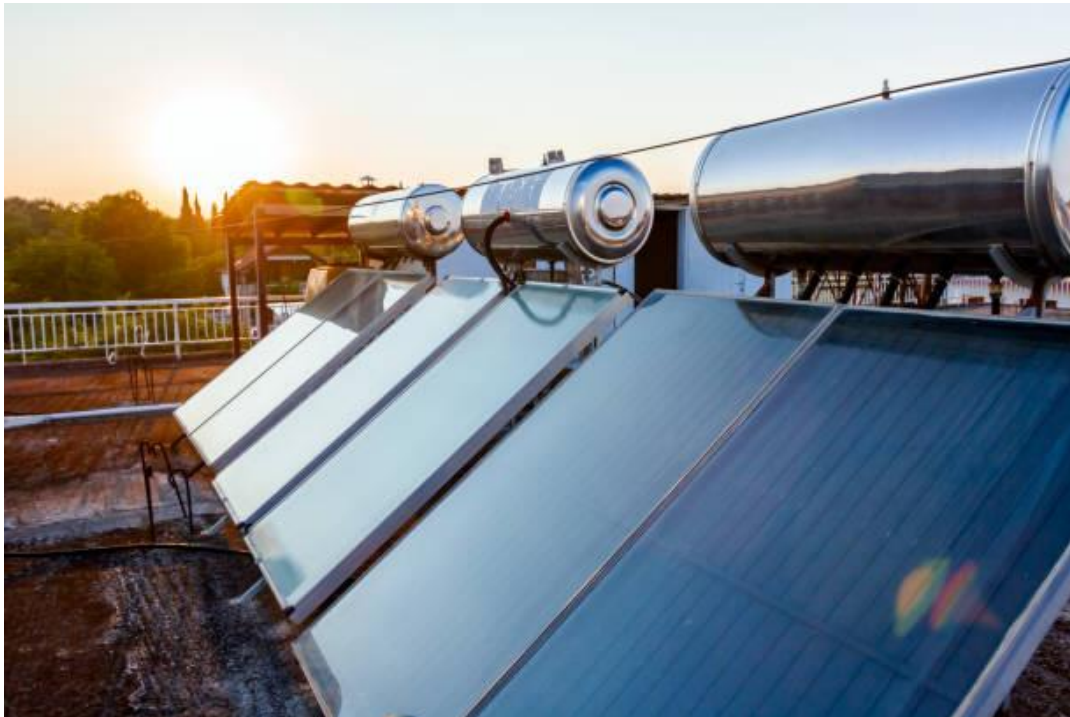
Figure 1.20: Domestic Water Heating (Photothermal Systems)
